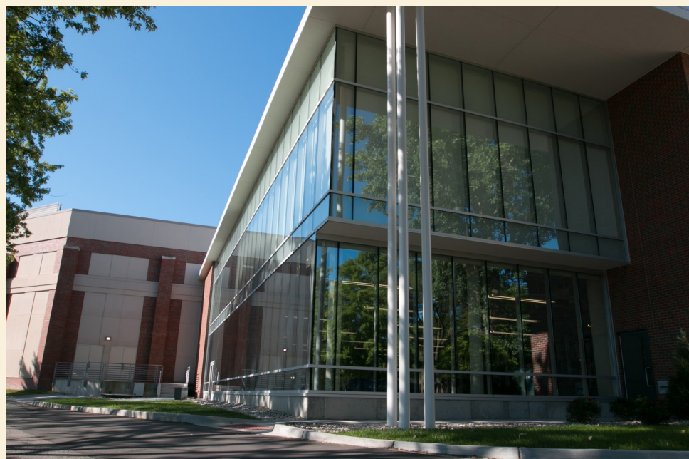
The expansion is a visually appealing two-story glass structure that faces the Fred Meijer Heartland Trail and Wright Avenue.
